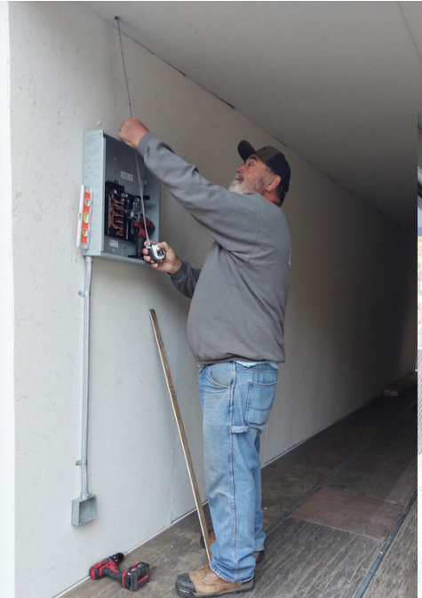
Slim, from Two Ton Electric, installs the electrical panel
