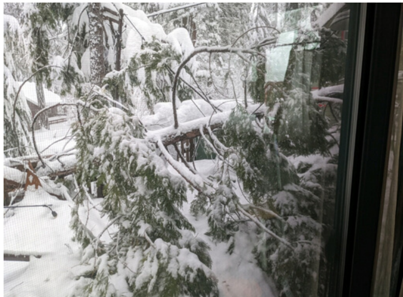
Storm damage in Twain Harte
