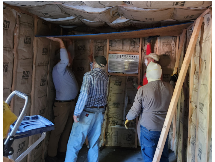
Ed, Mike, Bob, and Matt install sheathing over the insulation
