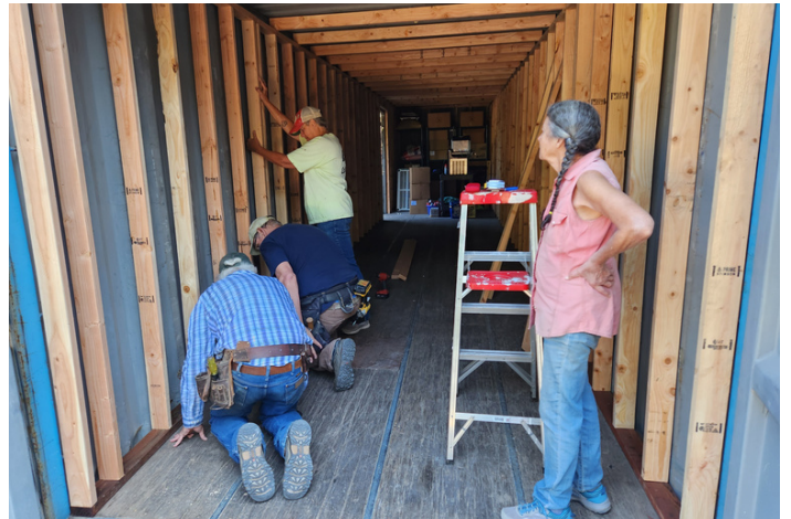
Mike, Bob, and Margaret install framing, while Lise looks on
