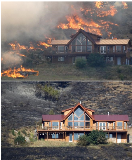
Ember Damage, but Building Saved
