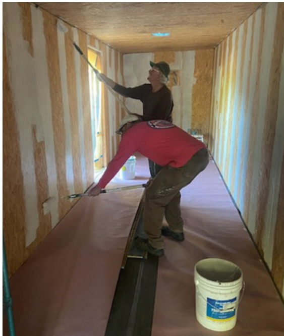
Bob Schreiner and Mike Mandell paint the interior of the container
