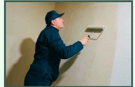
All shifts have been working hard on the sauna room.
