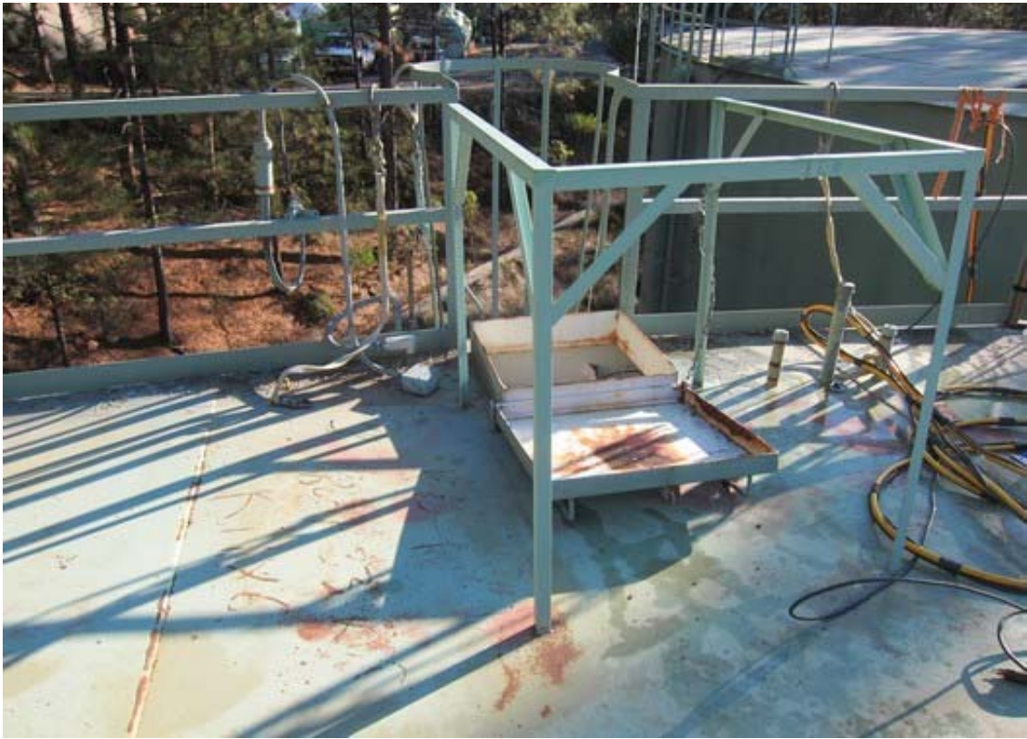
MG#2 Existing roof hatch, guardrail and appurtenances.
