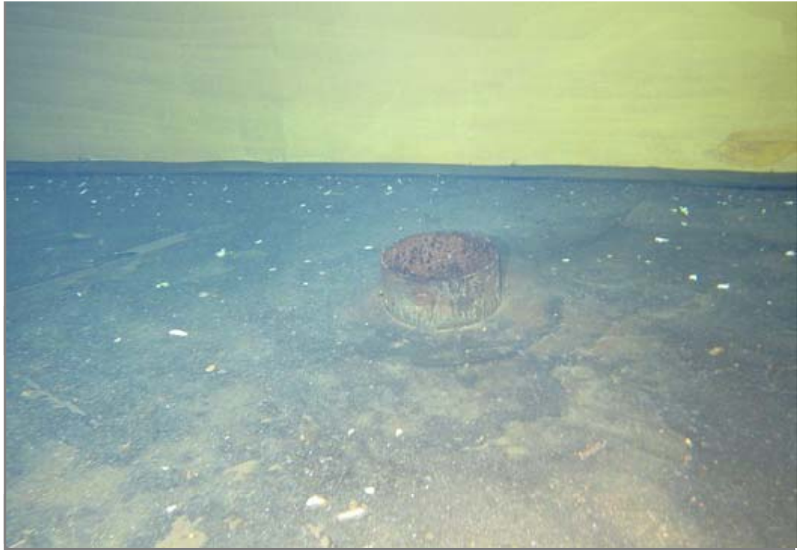
Interior bottom with the outlet penetration.
