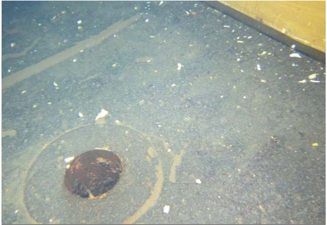
The drain is located approximately 4 ft. from the shell.
