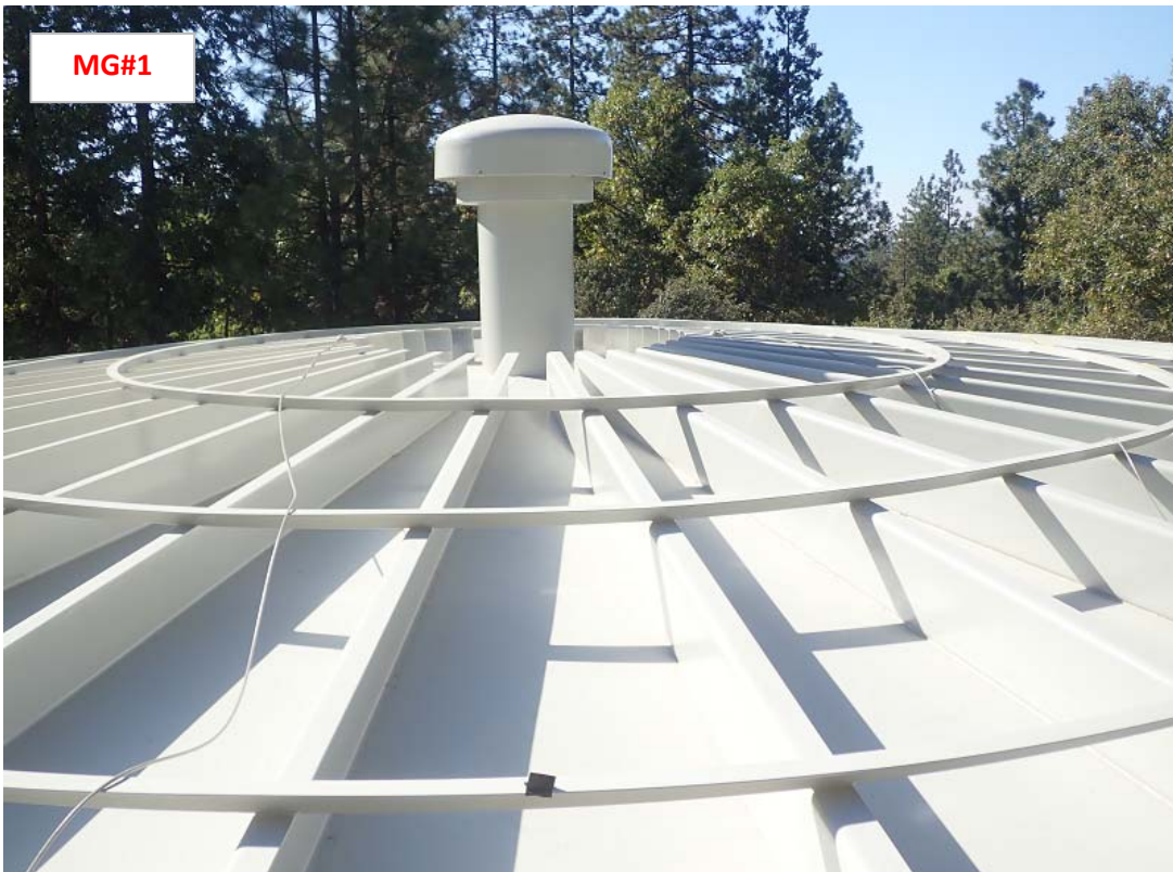
View of exterior roof of previously rehabilitated MG#1. The new roof, vent and guardrail on this MG#2 Rehabilitation project is to be similar.
