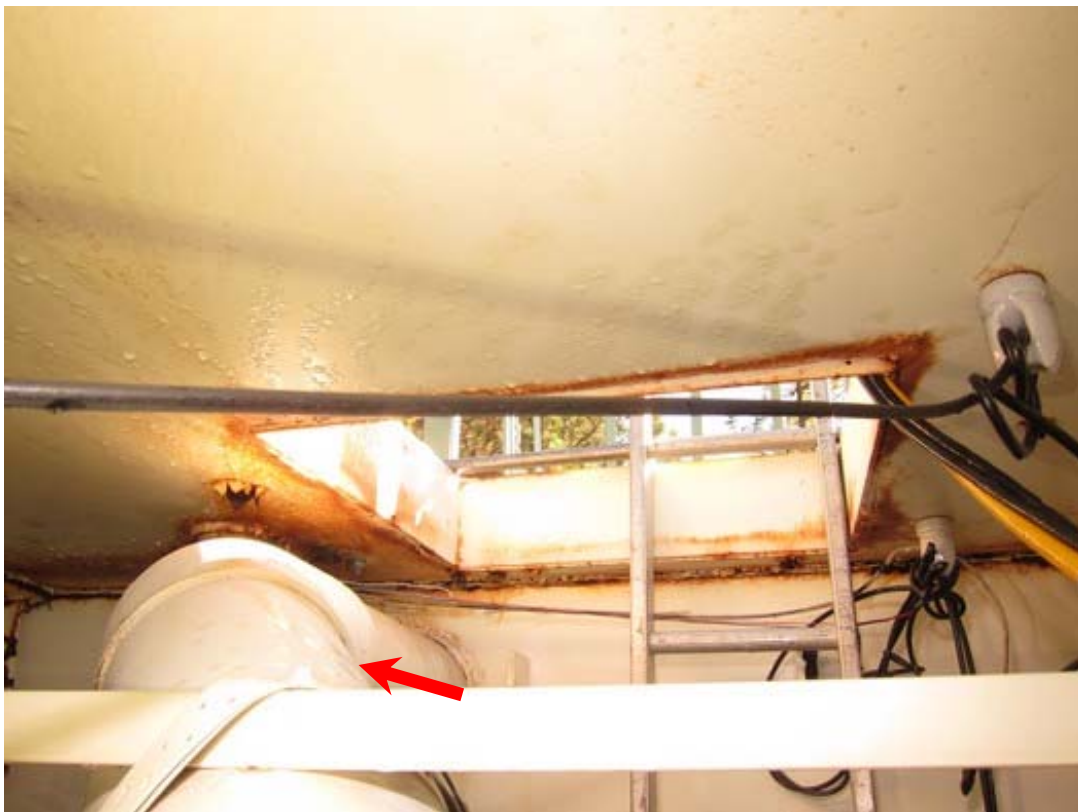
Existing PVC in high inlet pipe on MG#2 that will require protection during work and support from the new roof.
