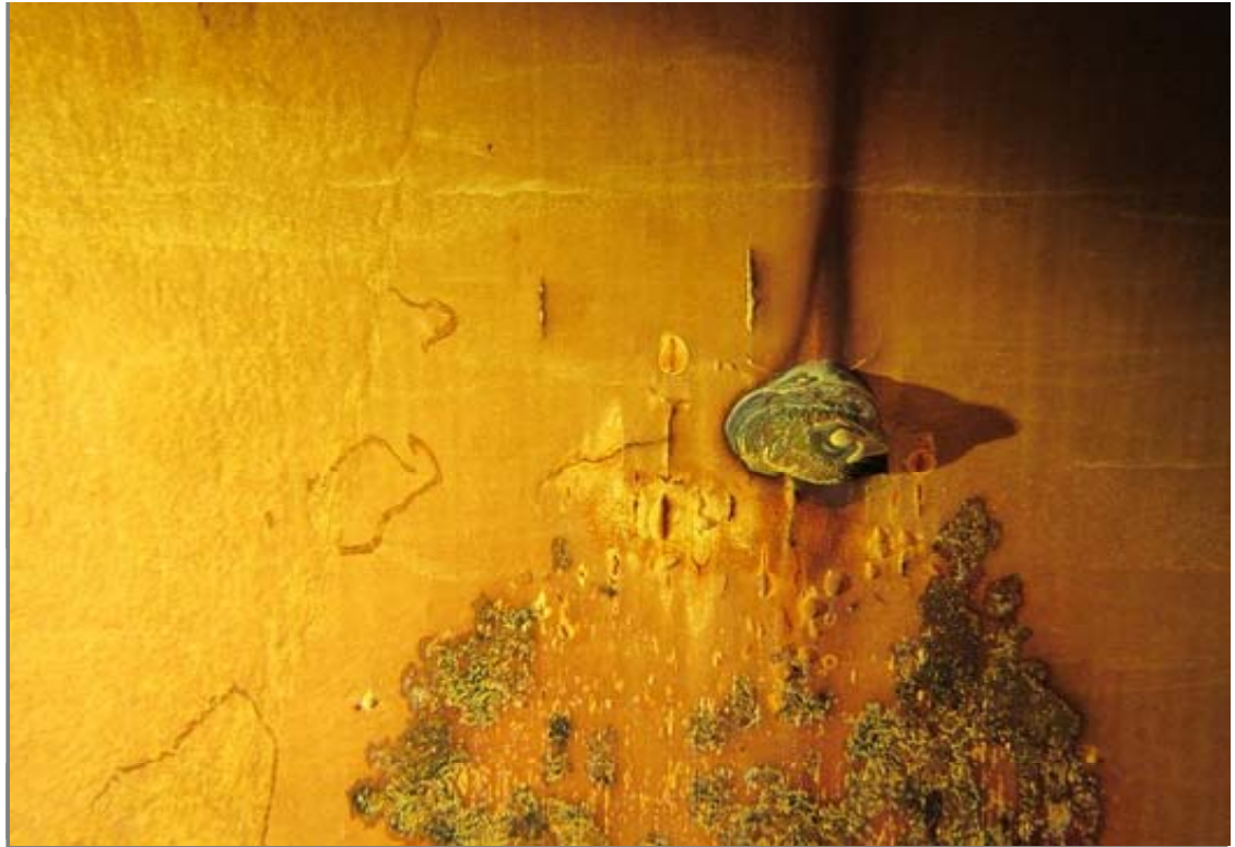
Interior shell in the submersion zone near the manway in quadrant 1. The coatings are cracking and corrosion is present.
