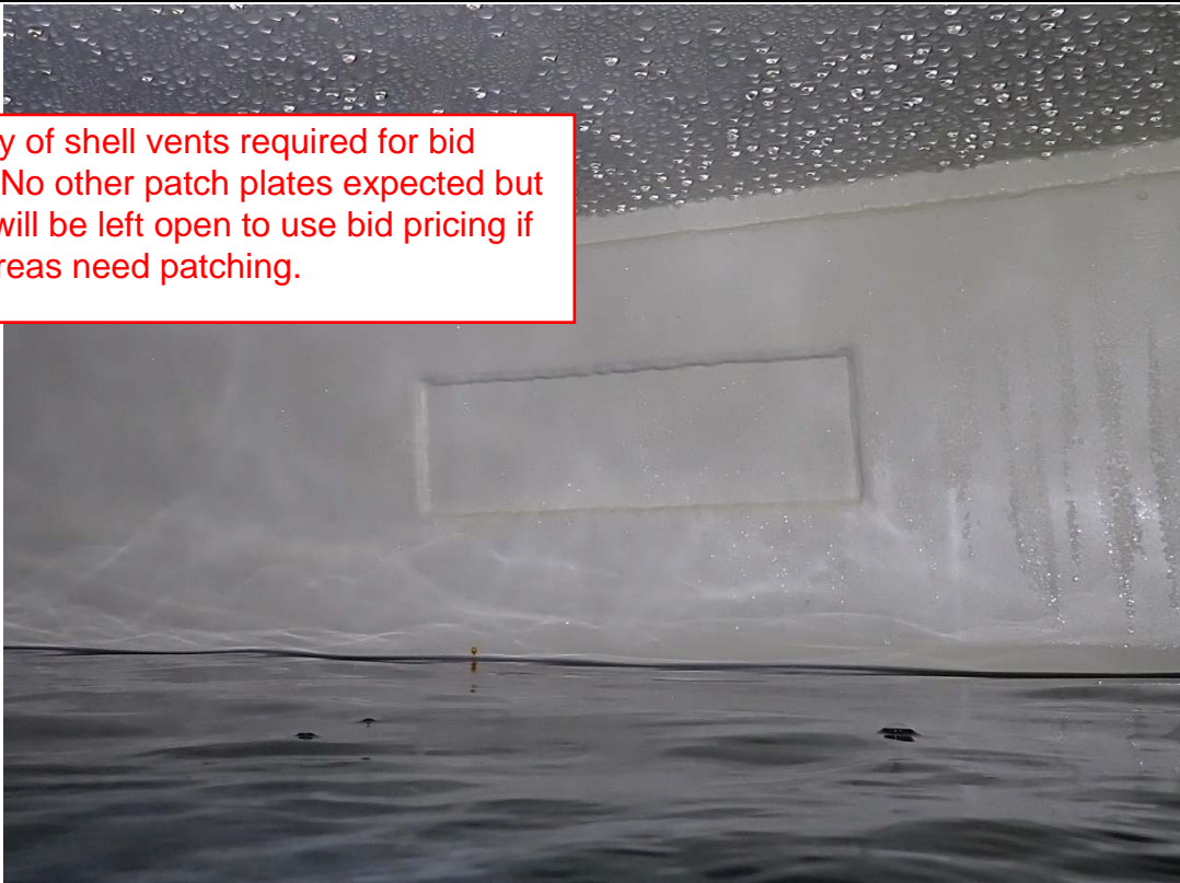
View of acceptable shell vent closure.
