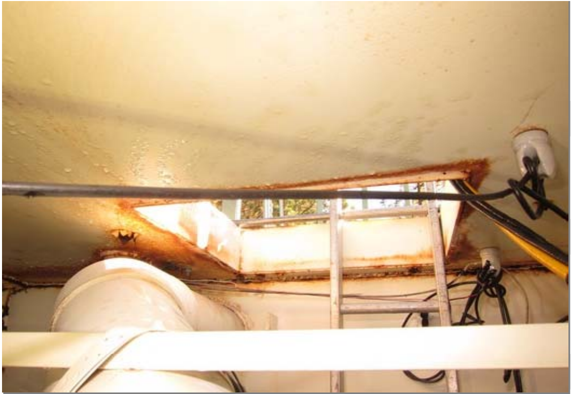
View of the roof hatch from the interior. The diver's entry ladder is visible.
