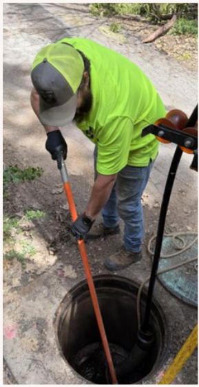
Routine sewer jetting & manhole inspections work.
