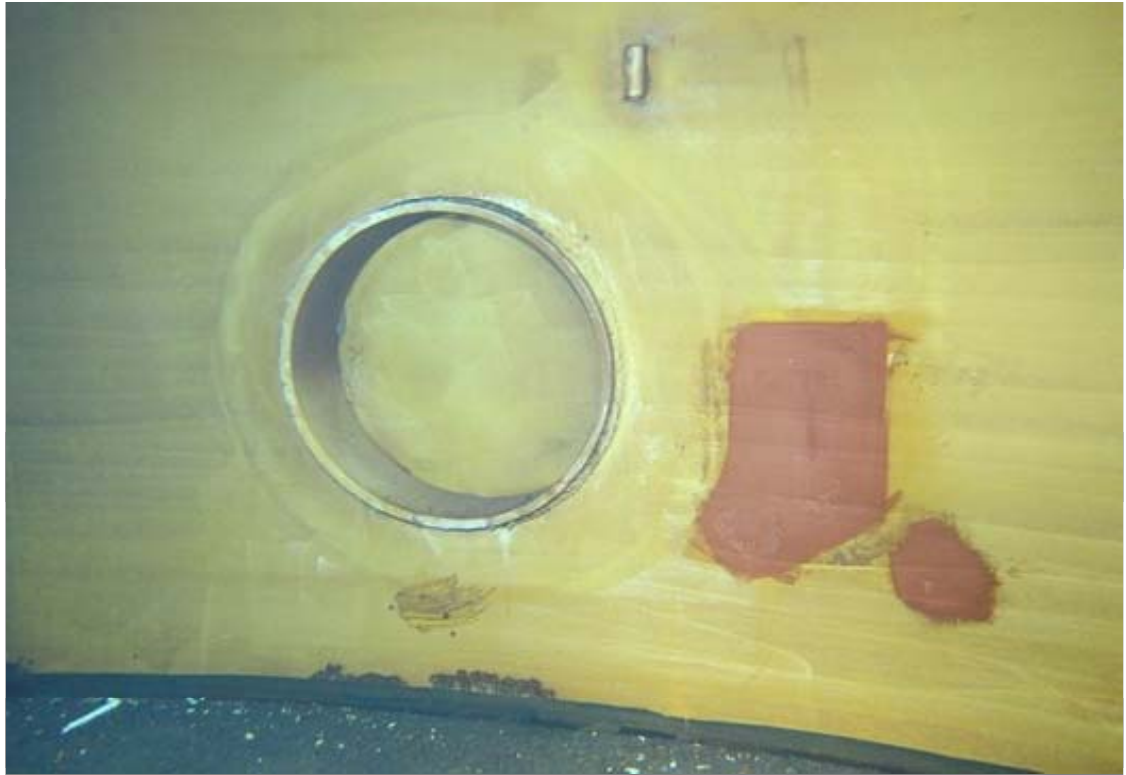
Interior view of the shell manway near quadrant 3. A spot repair is visible to the right and some significant corrosion is present below the manway.
