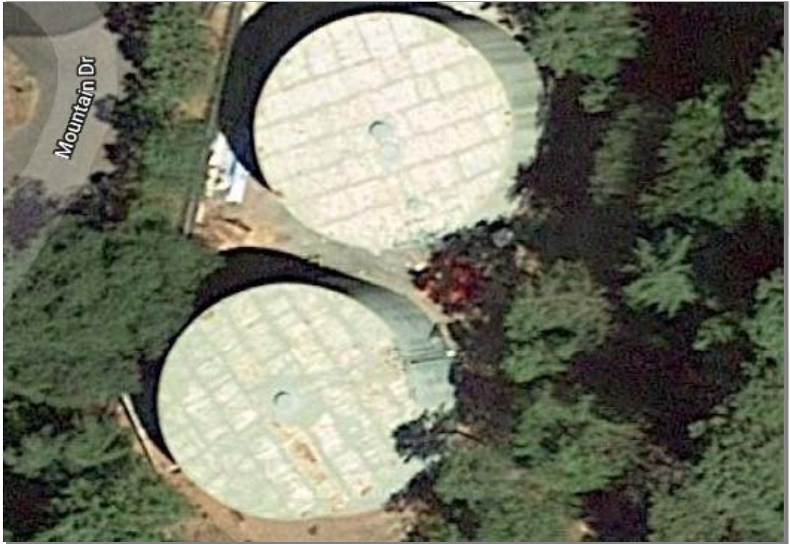
Plan view of tanks and site (courtesy of Google).
