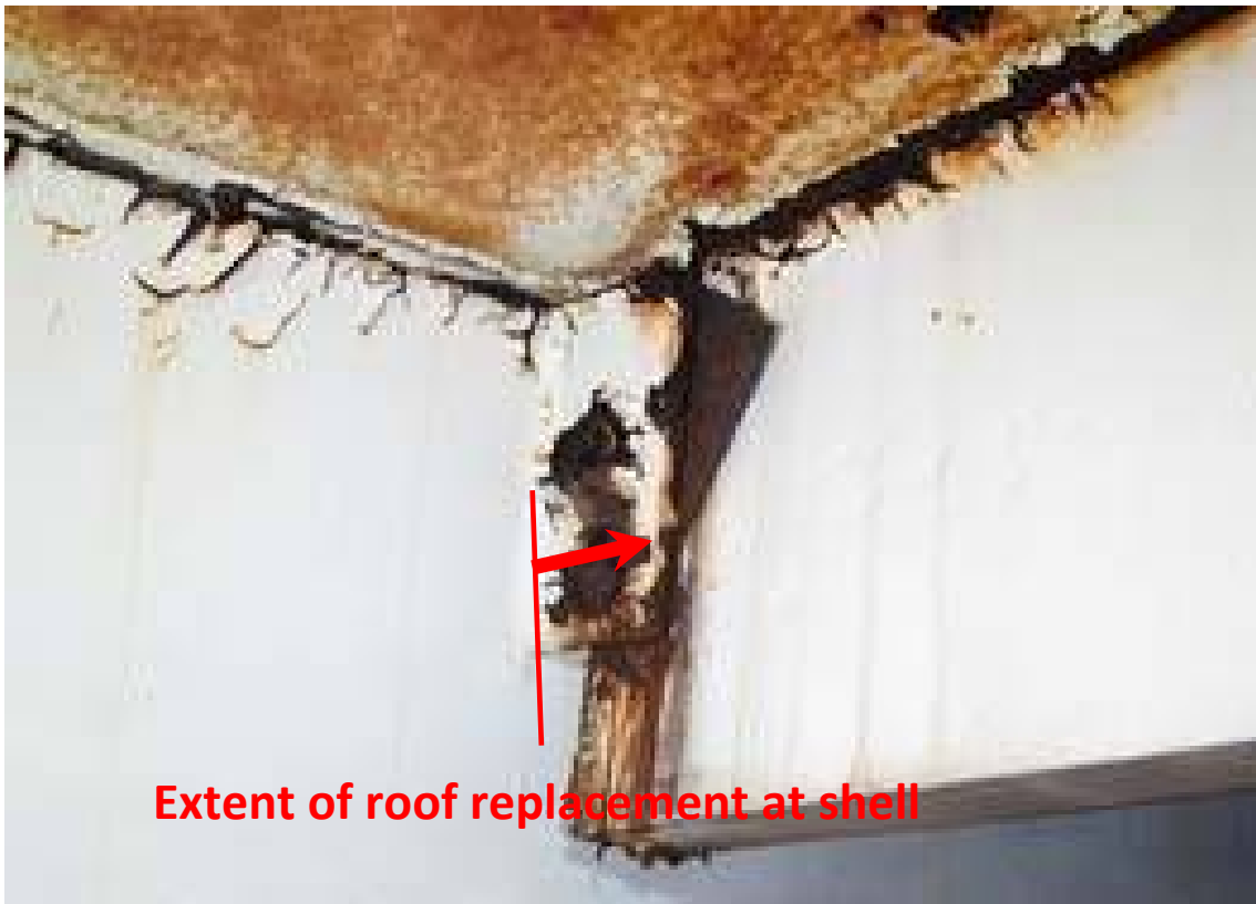
MG#2 existing rafter and shell clip and extent of roof replacement at the shell.
