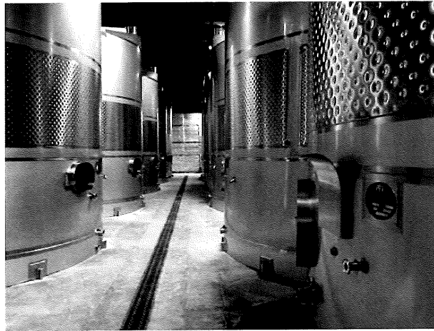
Paris Valley Road Winery Paso Robles, CA
