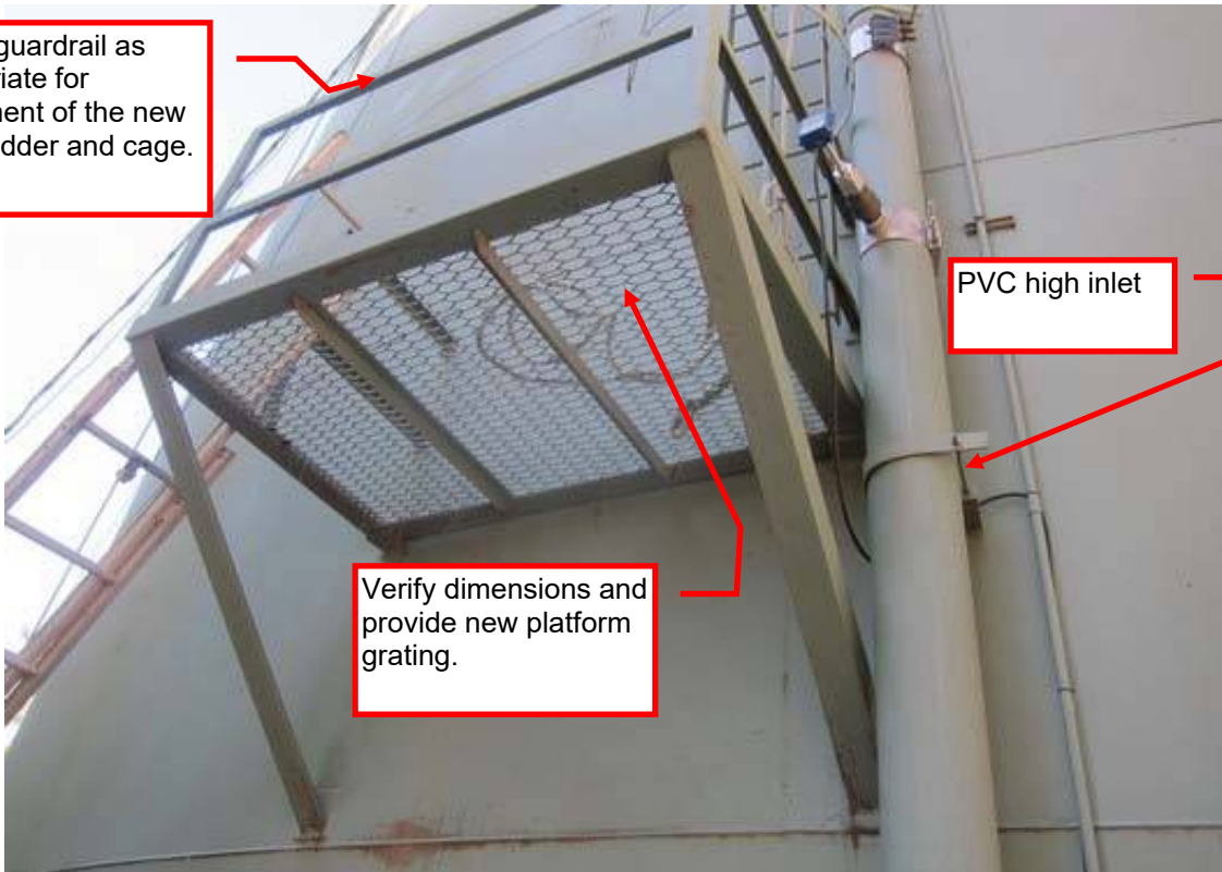
MG#2 Existing ladder platform. A new low section of ladder to the platform and appropriate additional guardrail and new grating on the platform are part of the scope of work.
