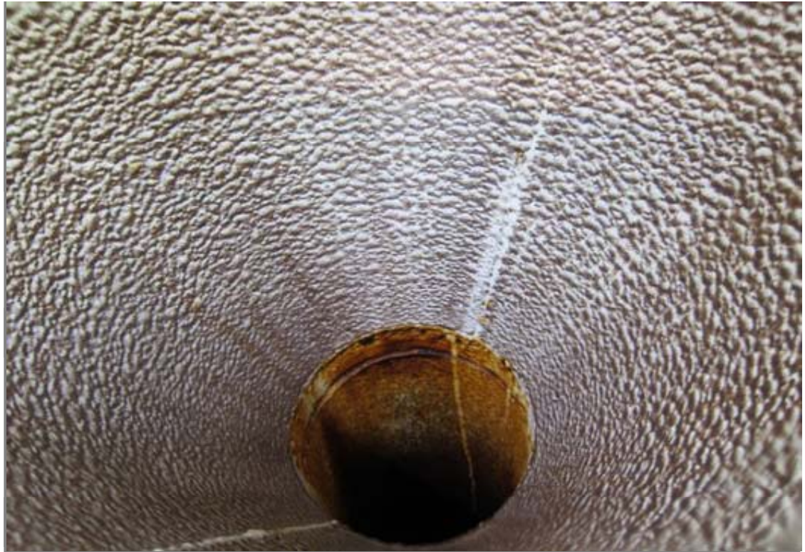
Interior of the overflow weir.
