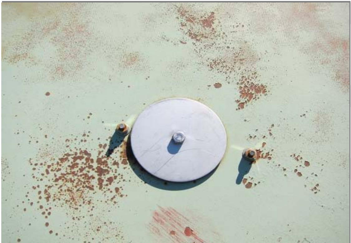
Typical view of a cathodic protection hand hole cover in good condition as viewed from the exterior roof.
