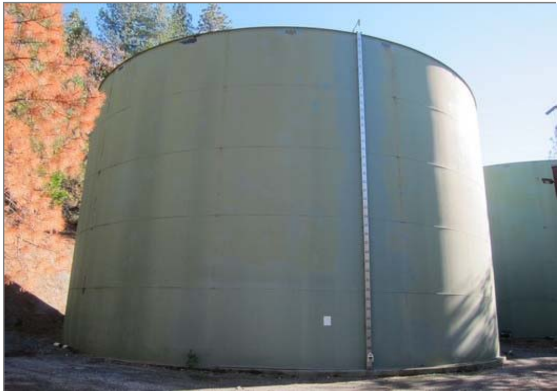
Overall view of the MG #2 Tank.
