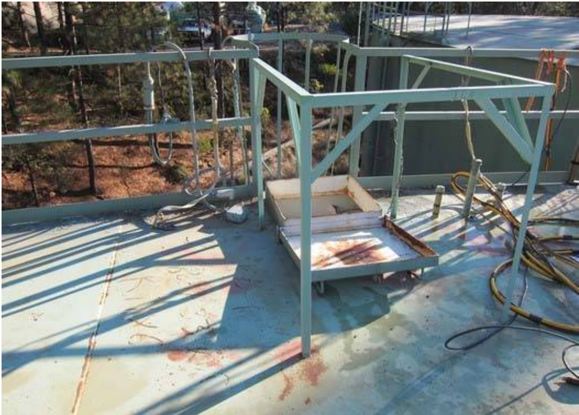
MG#2 Existing roof hatch, guardrail and appurtenances.
