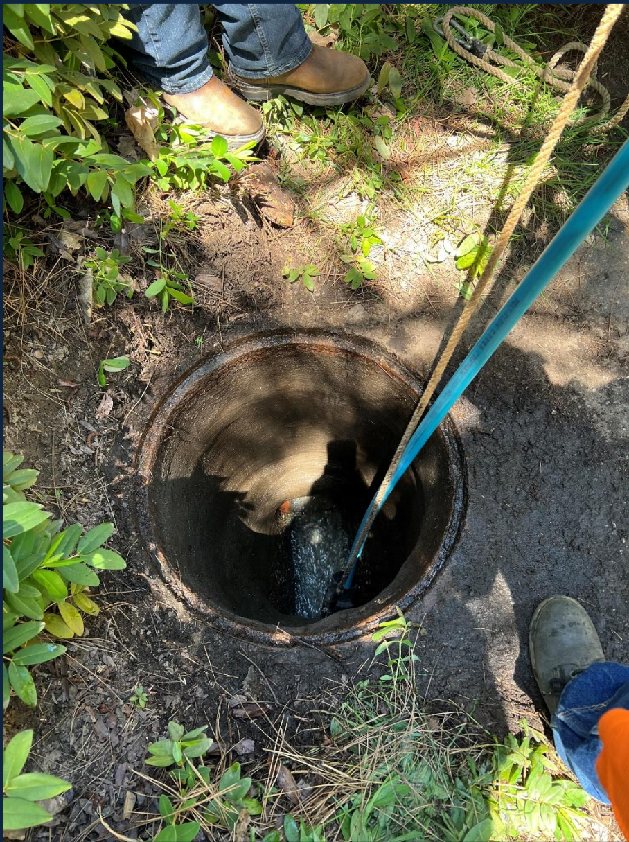
Top Left: Sewer jetting along the lake bench (south side of lake)
