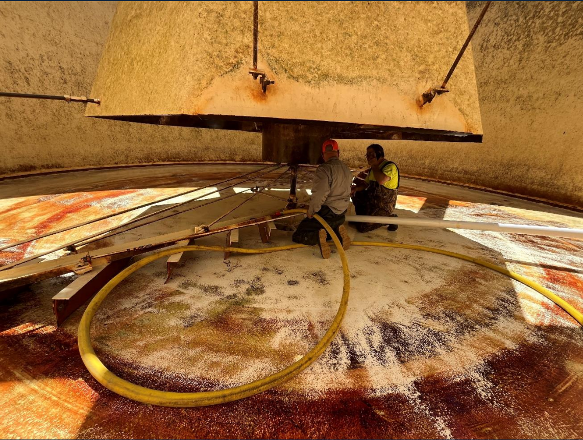
Top Left: Biannual clarifier draining, cleaning and repairs.
