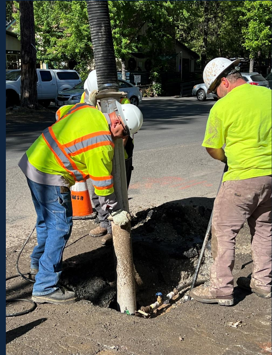
Top Center: Identifying all utility locations at Vantage Pointe ahead of parking lot project.
