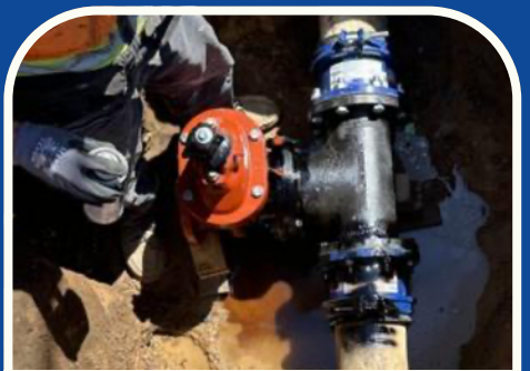
Tie-in for the Manzanita Ct. waterline upsizing.
