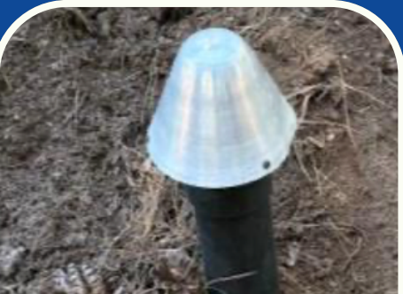
Sewer failed cleanouts from the smoke testing inspections have been repaired.
