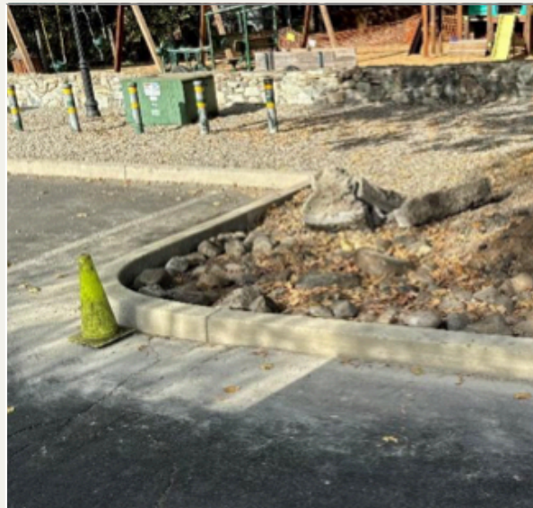
Completion of the curb repairs at Eproson Park
