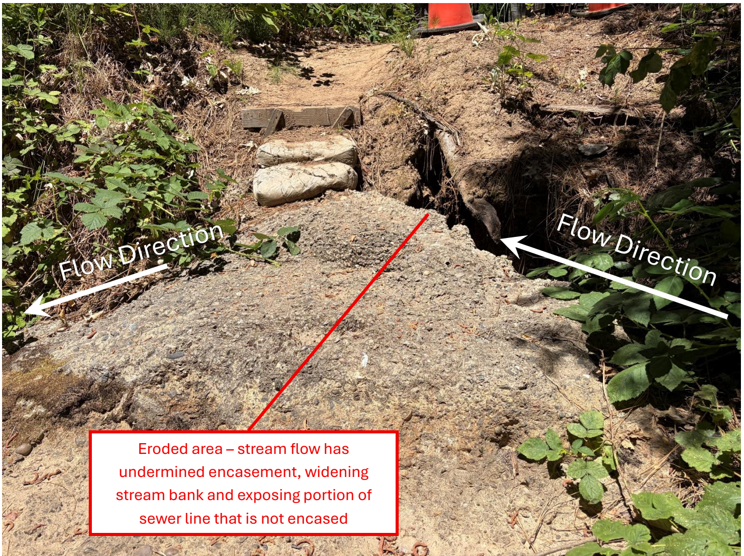
Undermined and eroded encasement. End of encasement used to be completely covered by dirt within the bank.
