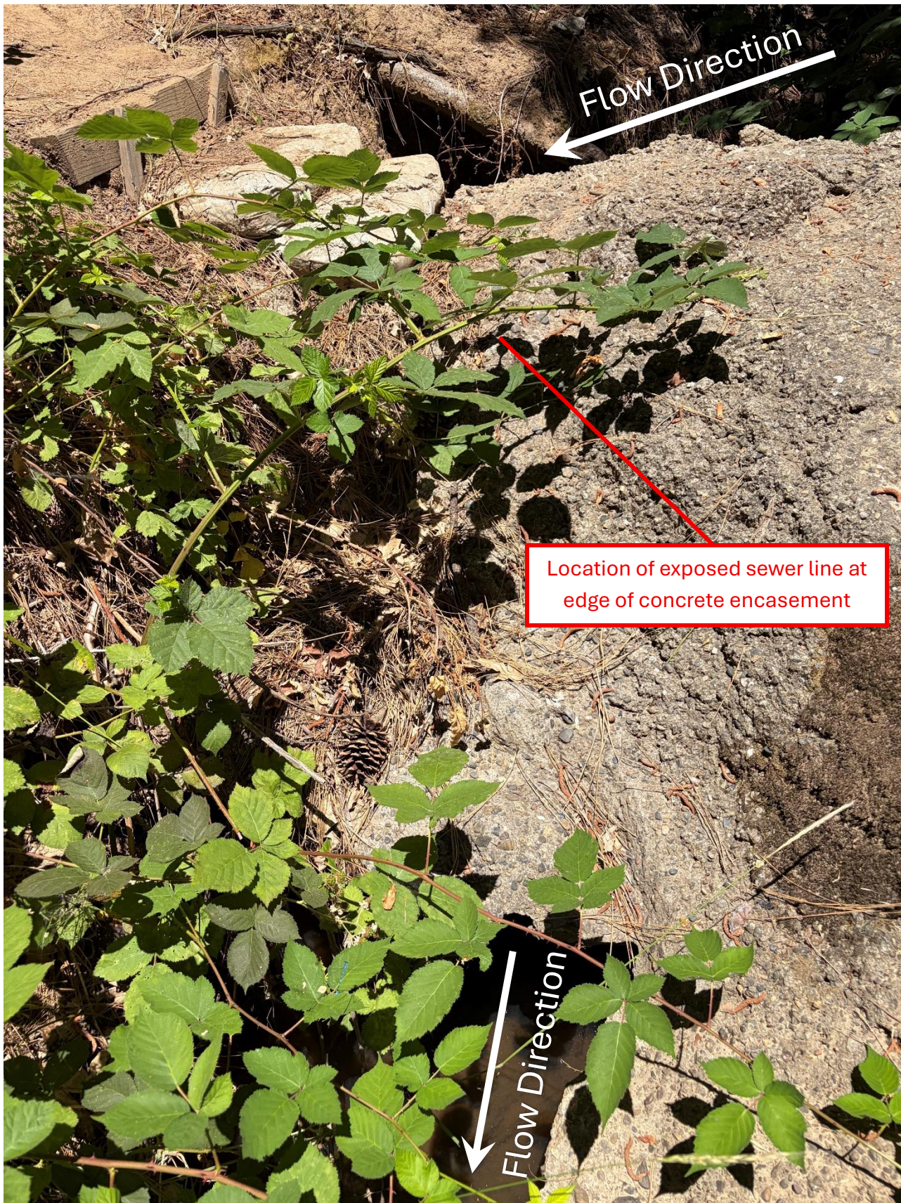
Undermined and eroded encasement. End of encasement used to be completely covered by dirt within the bank.
